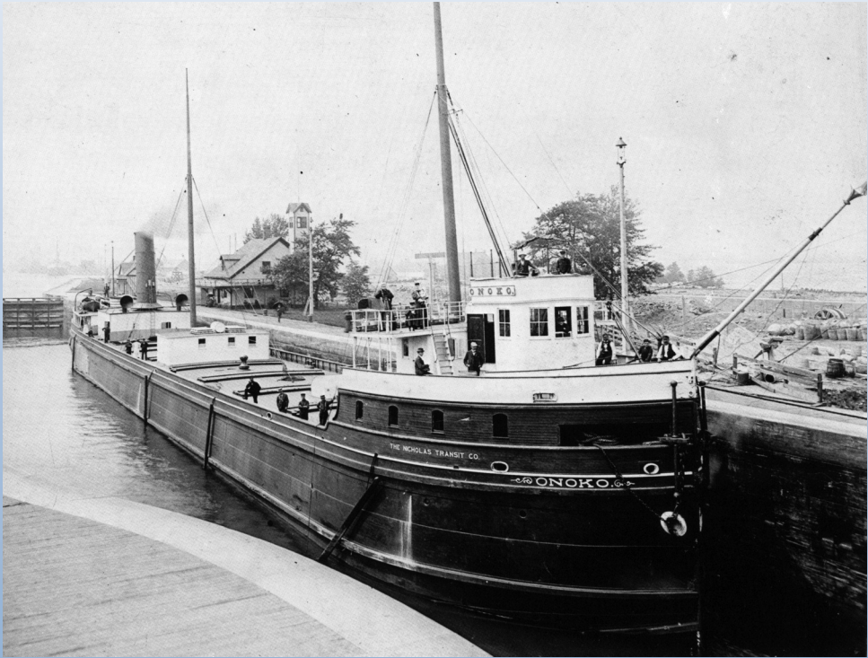
The Onoko , one of the earliest (1882) iron hull, steam-powered, water-ballasted ships on the Great Lakes.
